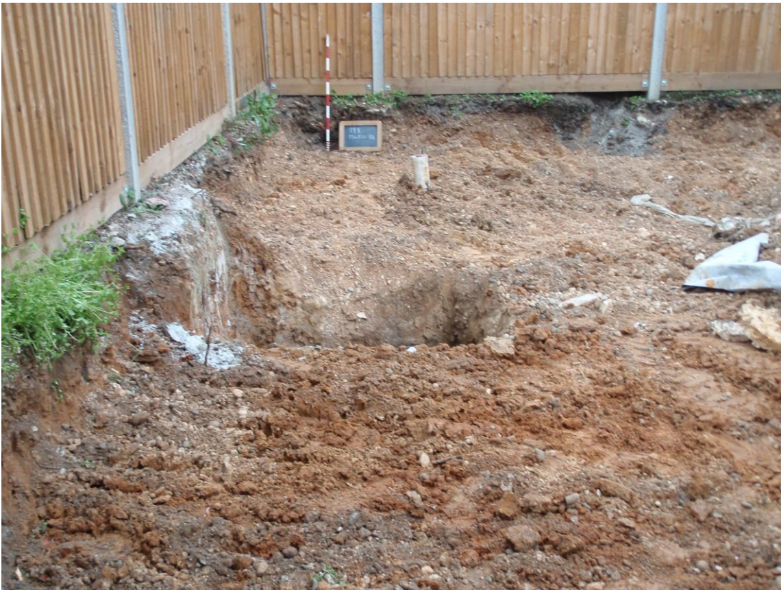
Plate 5. Extent of trench (looking NE)
